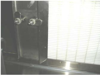
STEP # 5 - FILTER JACK LOCKING TABS SHOULD NOW BE PENDICULAR TO KNIFE EDGE AND FILTER FRAME
