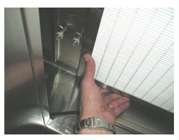
STEP #3 - PUSH FILTER FIRMLY FROM EDGE TO SEAT FILTER \* CAUTION DO NOT PUSH ON FILTER MEDIA!\* MEDIA OF FILTER IS EASILY DAMAGED
