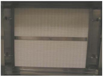
PROPERLY INSTALLED GEL SEAL FILTER WITH FILTER LOCKING TABS
