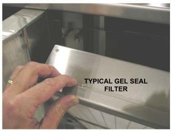
STEP #2 - POSITION FILTER INTO OPENING OF UNIT \* BE SURE FILTER IS CENTERED IN OPENING\*
